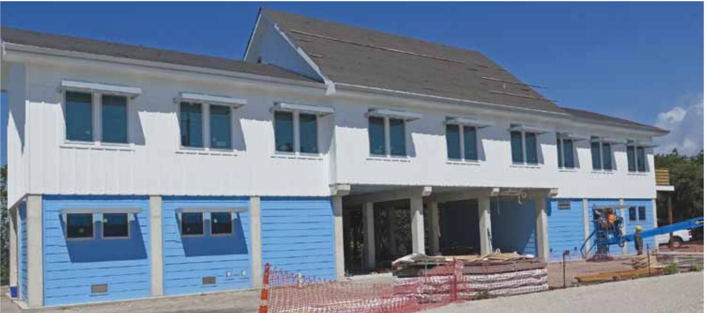
*The exterior of the new Marine Lab at Tarpon Bay has been painted, and the gutters and window shades have been installed. Much more work is happening inside the Lab. Electrical and plumbing rough-ins were finished in February and drywall started in March.*
