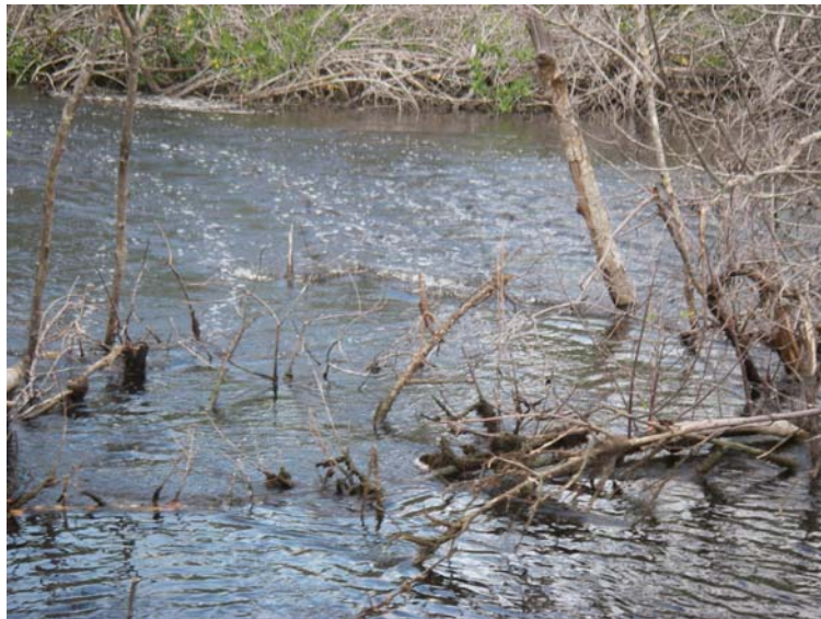
January, 2006 – 35 foot x 7 foot depth breach develops at West end of the lift dam
